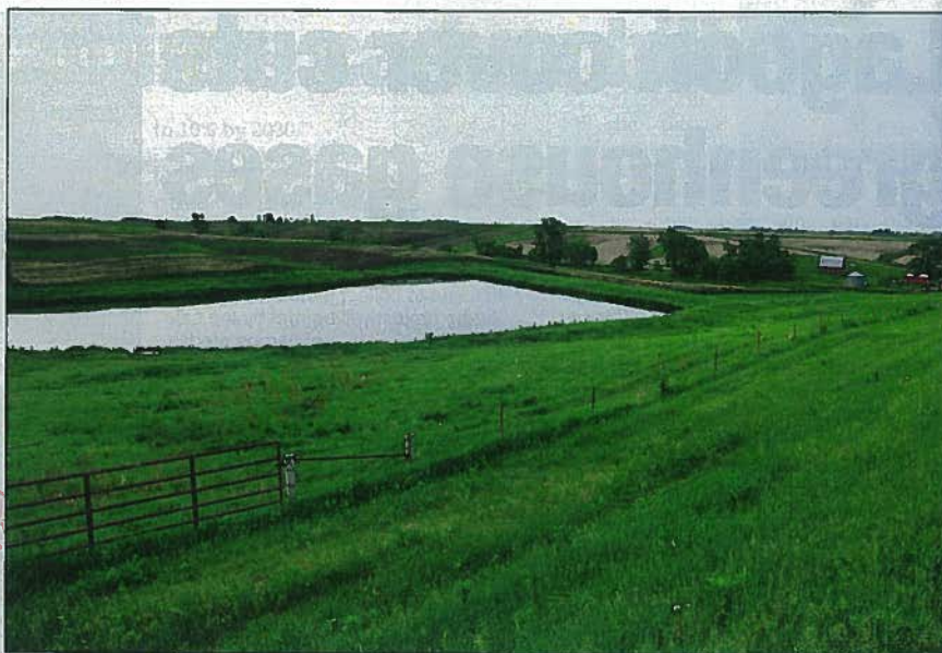
POND BUILDING ESTIMATES: A detailed, accurate estimate of costs to build ponds like this one can be made in the NRCS office in less than 15 minutes. New computer software and LIDAR elevation data is now available in some states.
