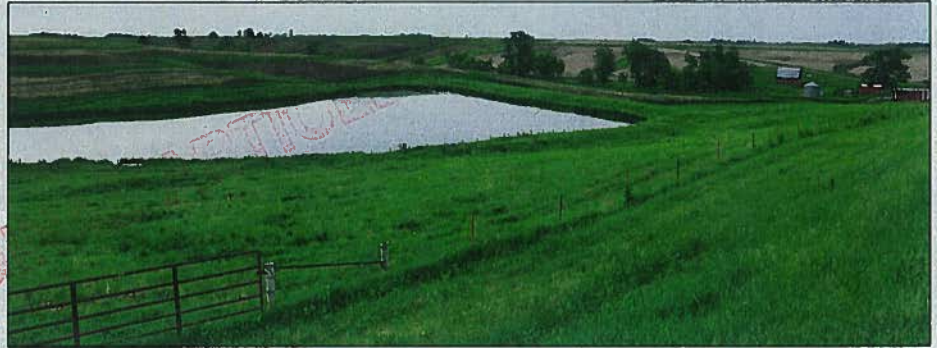
POND PRICES: A detailed, accurate cost estimate to build ponds like this one can be made in the NRCS office in less than 10 minutes, with new computer software and LIDAR elevation data.
